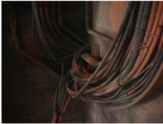
Figure 4: Example of poor cable installation
